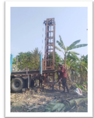
Drilling a Well
